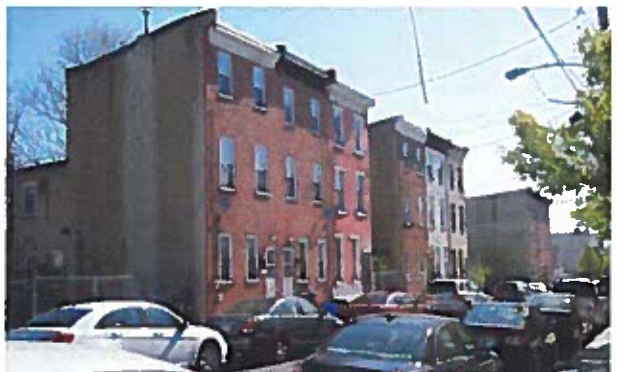
View of the existing rowhouses on the southeast corner of the site
