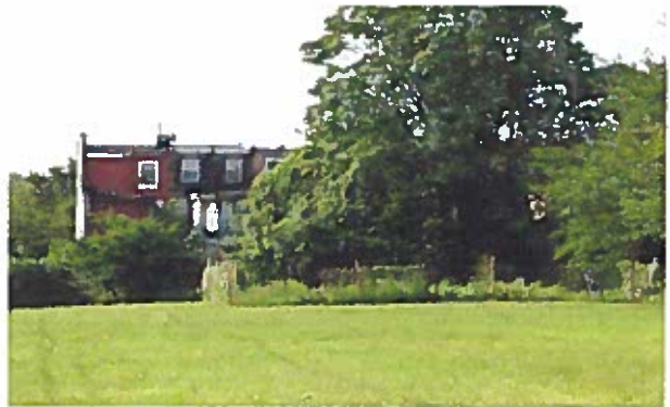
View of the rears of the rowhouses on the south side of the site
