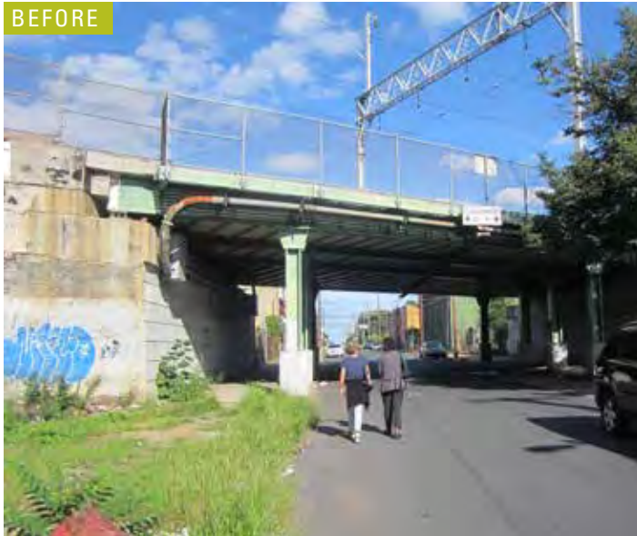
Corridor Improvements on Susquehanna
