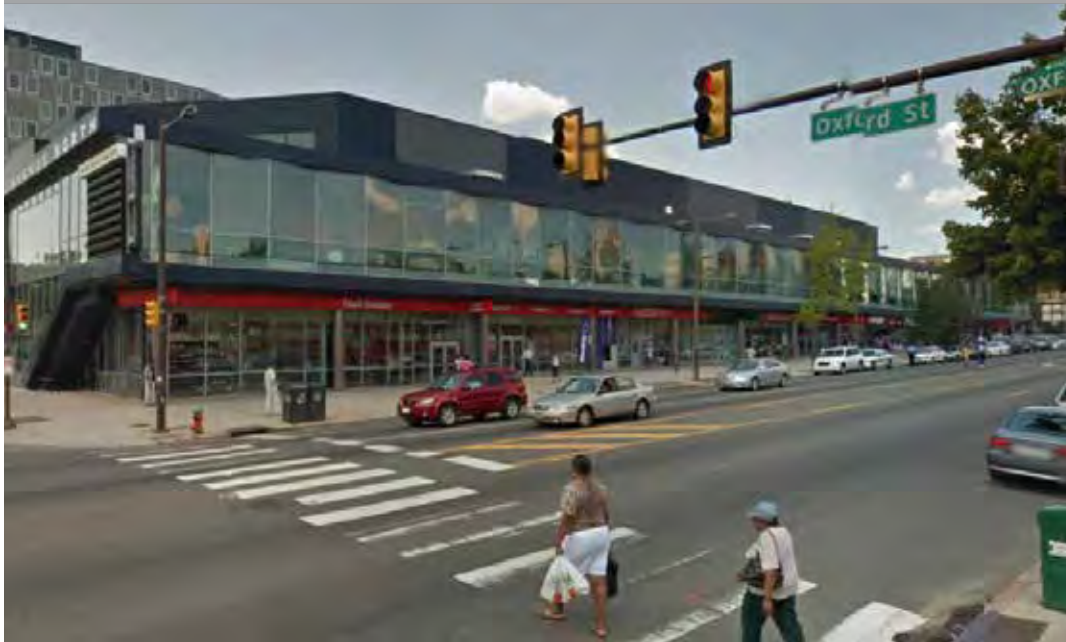
Completed in 2006, Avenue North is one of the hallmarks of Broad Streets rebirth. The 66,000-square foot retail center features The Pearl Theatre (27,000-square foot, seven-screen movie theatre) the first cinema to be developed in North Philadelphia in nearly 60 years.
