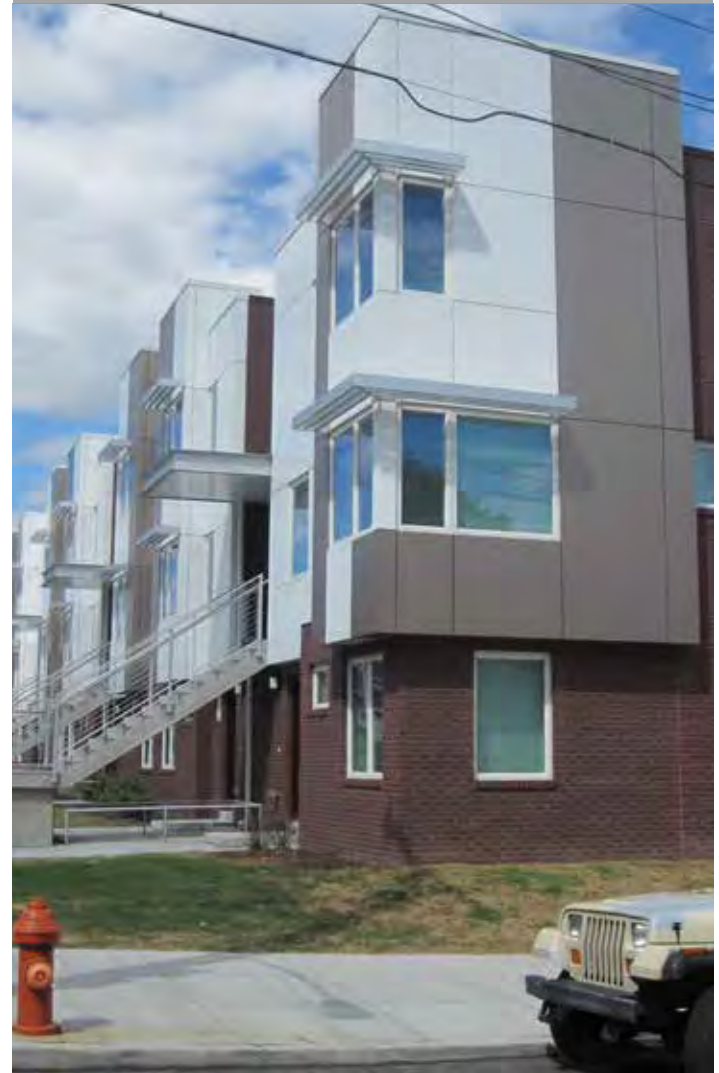
The new Norris Apartments replaces the 1950s high-rise building with the PHA's first LEED certified building. The new complex features 51 units in a mix of walkups and townhomes. The new homes have solar hot water panels on the roof, Energy Star windows, equipment and appliances, low flow plumbing fixtures, and compact fluorescent light (CFL) fixtures.
