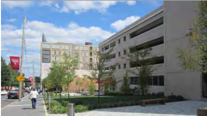
The new $25.4 Million garage provides 1,100 parking spaces and retail on Berks Street connecting to Temple University's Polett Walk. The Kardon/Atlantic Terminal Building (background) is listed on the National Register of Historic Places and includes apartments and office space.
