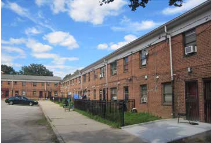
Existing Norris Apartments
