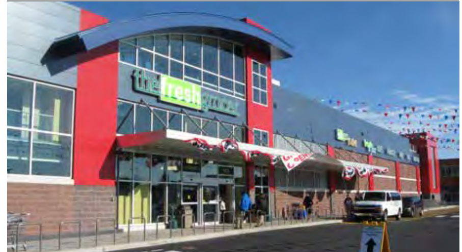
Progress Plaza is the nation's oldest African-American owned and operated shopping center. After going through significant vacancy, the shopping center was rebuilt in 2009 to include a $15 million, 46,000 square foot, full-service supermarket. The Fresh Grocer financed in part by funding from the state Fresh Food Financing Initiative brings affordable, healthy food choices to the community, as well as 272 jobs many filled by residents from the surrounding neighborhood. (Source The Reinvestment Fund)
