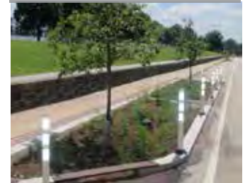
Stormwater bumpouts installed by PWD on Queen Lane in East Falls.
