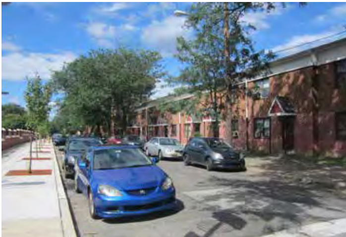
Existing Norris Apartments
