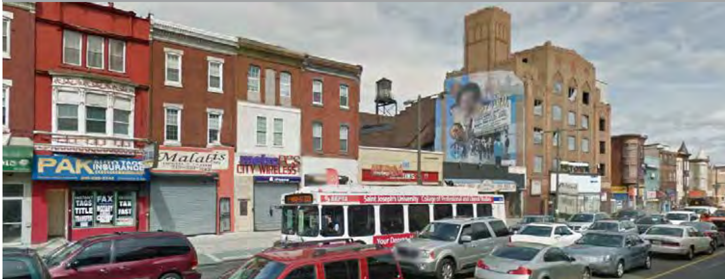
Broad Street is being targeted for comprehensive improvements through a collaborative effort by government, non-profit, institutions and private developers. The goal is to reestablish North Broad Street as a vibrant urban thoroughfare that supports arts, culture, and entertainment, institutional and commercial development.
